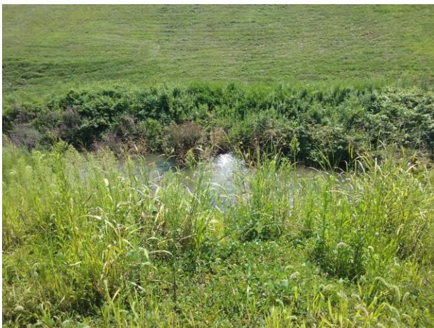
Photo 5 – Typical view of the downstream slope showing at the discharge pipe for the fly ash pond..
