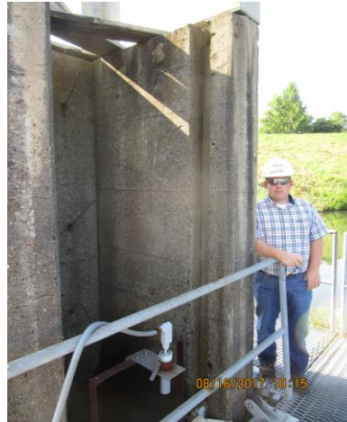
Photo 2 – Typical view of decant structure showing good conditions. Paul Hutchins is also depicted and participated in the inspection.
