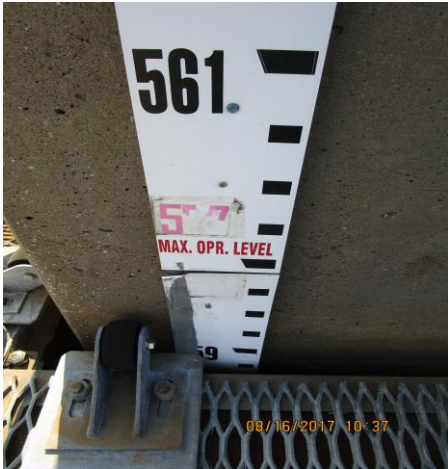
Photo 1 Typical view of staff gage denoting Max Operating Pool.
