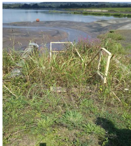
Photo 6 – A small area where excessive vegetation has grown along stairwell access.
