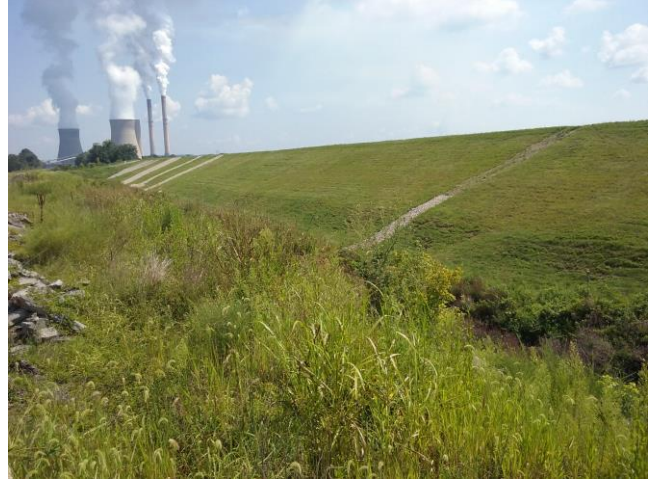
Photo 8– Typical view of the repairs to the seeps along the west embankment showing excellent conditions.
