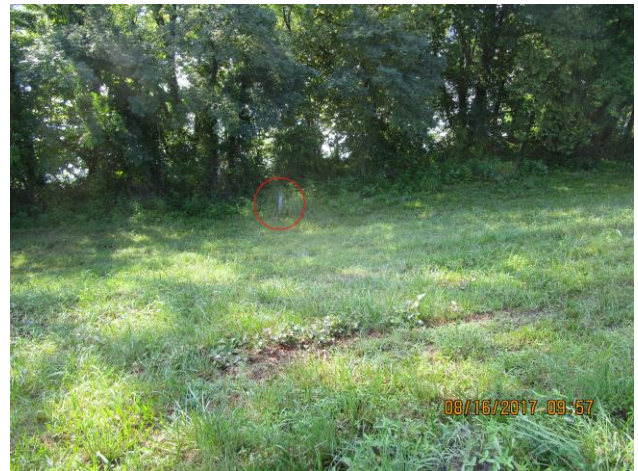
Photo 4 – Typical view of the downstream slope showing the location of the piezometer KC-1022 along the edge of mowed area.
