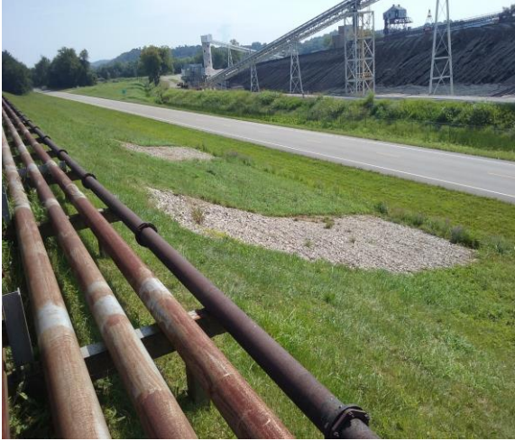
Photo 7 – Typical view of the repairs to the seeps along the east embankment.
