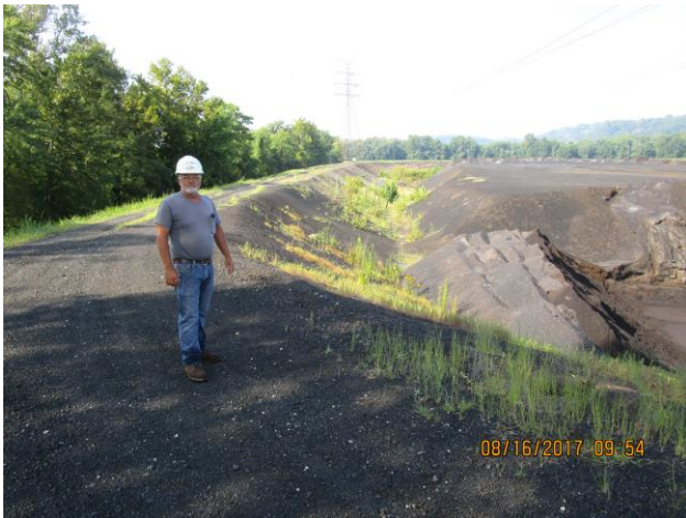
Photo 3 – Typical view of crest and embankment showing good conditions. Ken Stapleton is also depicted and participated in the inspection.
